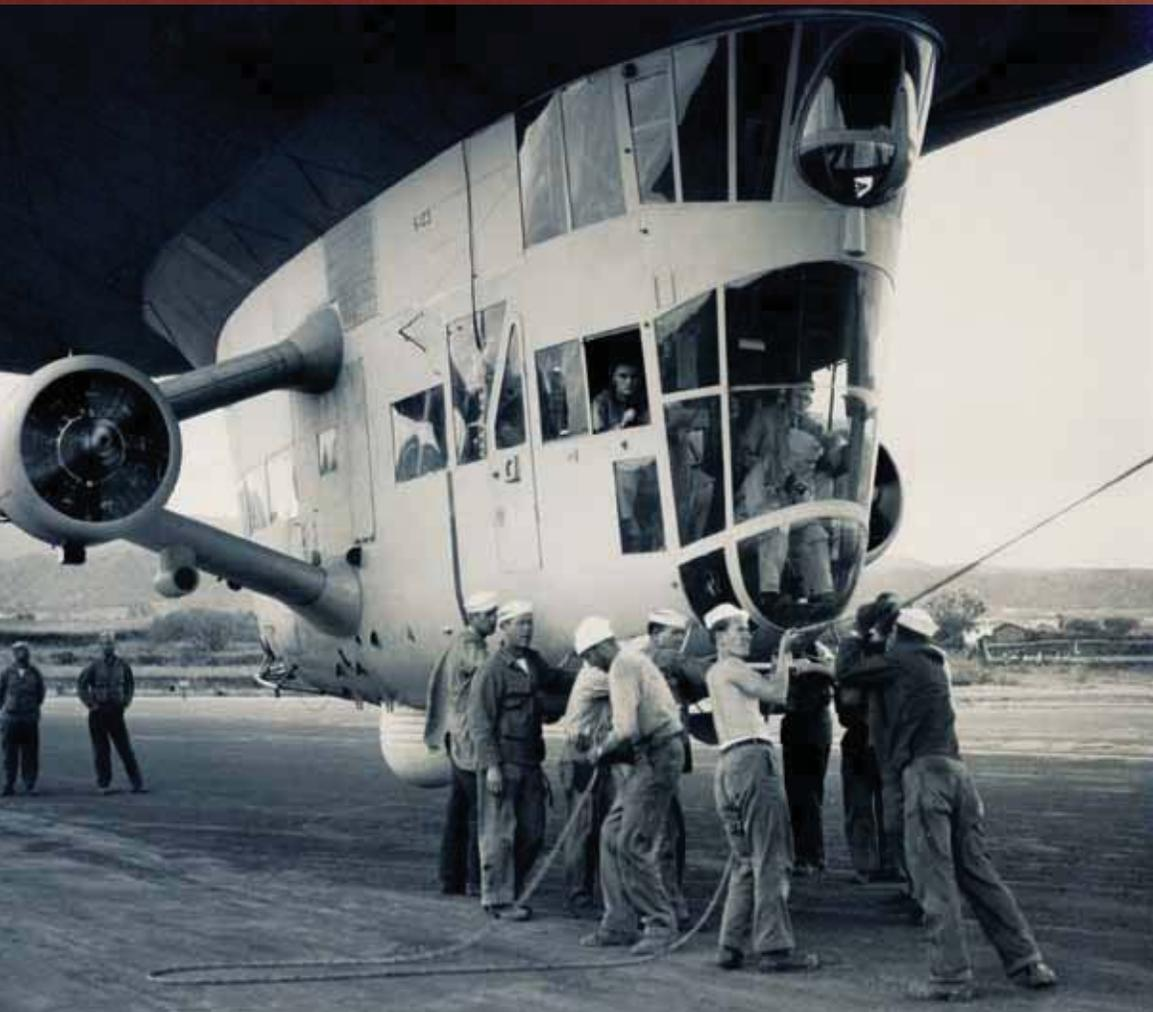
*K-123 was the first airship to take-off from Lagens Field on Terceira Island in the Azores on 31 May 1944. Lt. j.g. Homer Bly (pilot) manned the elevator (top right in the control car), Ens. Warren Ireland (co-pilot) manned the rudder (window, top left), and Ens. William Kaiser (co-pilot) took the forward lookout position. (Photo from William Kaiser)*
